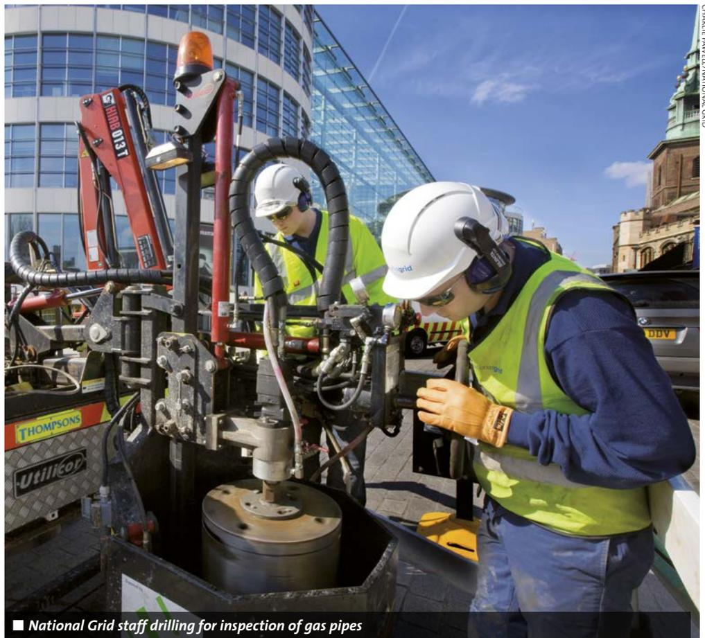
■ National Grid staff drilling for inspection of gas pipes
