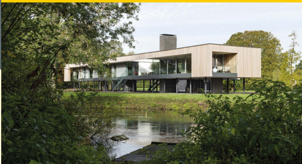
■ The Narula House, Berkshire: a flood-resilient design by John Pardey Architects (JPA) Image: nicoleengland.com (with permission)
