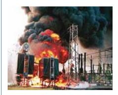
The direct cause of the incident was the failure of the mechanism in the tap changer leading to an electrical fault which caused the oil in the unit to ignite and explode.
