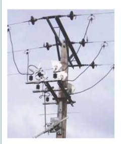
Following the issue of the Permit to Work, and some hours later, the control engineer closed the auto re-closer, believing he was energising up to the open isolators only. This resulted in one phase of the section of network covered by the permit to work being energised.
